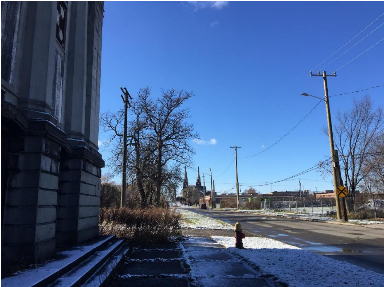
Image 4: Looking away from the church property past E Canfield St side of the abandoned church building. Some pavement removal is recommended here between the sidewalk and the steps of the building.
