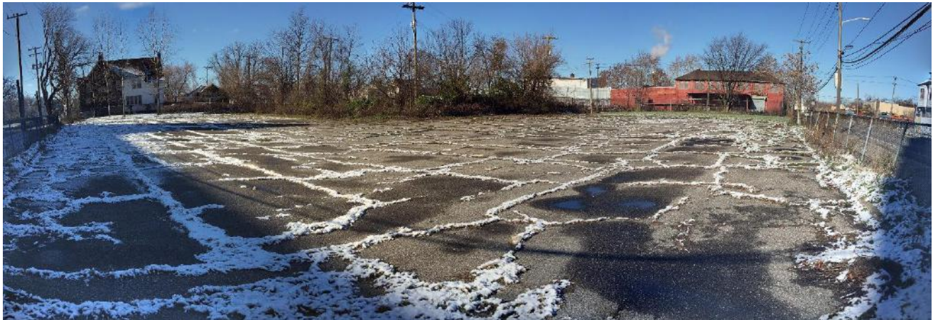
Image 1: The church-owned parking lot across from the church building. Practice 1 is proposed surrounding the existing catch basin in the center of the lot, to intercept runoff from the parking lot.
